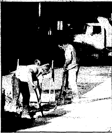
WORK CREWS took advantage of the sunny weather Tuesday to catch up on the 7th and North Main road construction.
